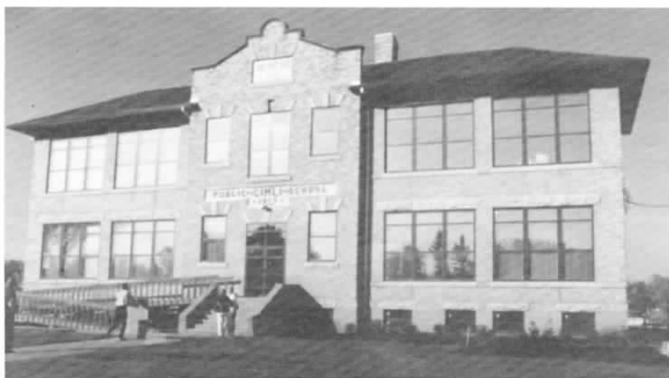
The school building, once attended by Leo Kristjanson, barely escaped the wrecker's ball a few years ago. Instead, it was completely rebuilt, with new windows, inside walls, flooring and lighting. An elevator, wheel chair accessibility and air conditioning were added to make it more functional. The place looks great. It houses the Town of Gimli offices, five other public offices, council and public meeting rooms, and a model classroom, circa 1920.
